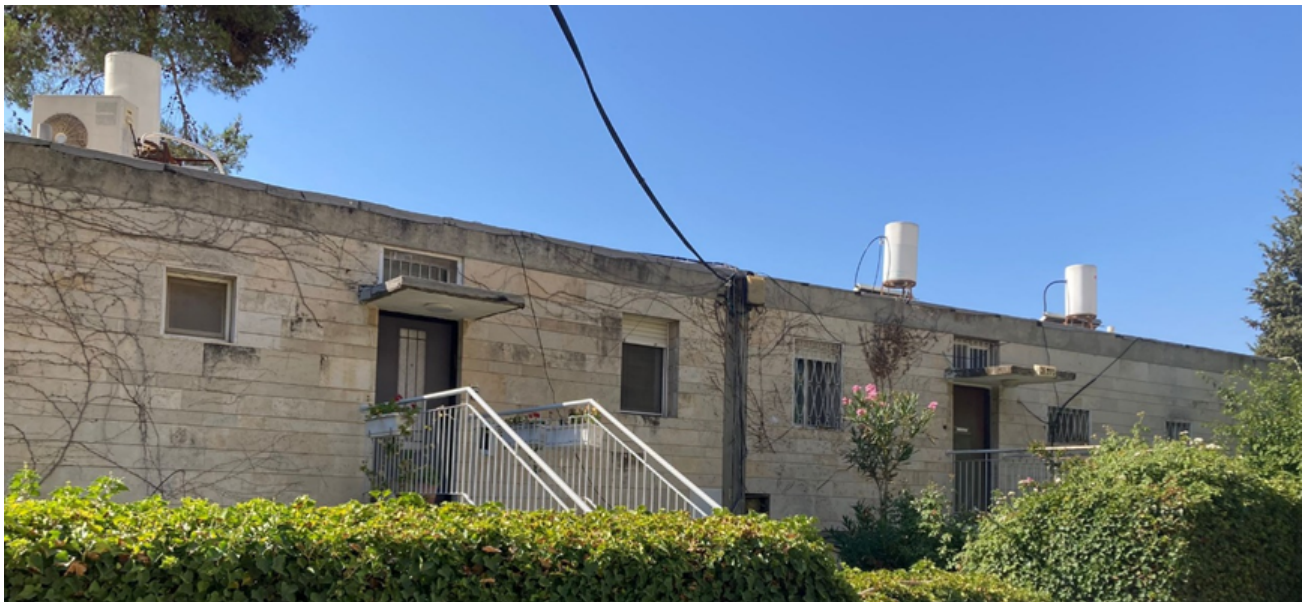
Figure 2: Adjacent Houses in the Neve Sha'anani Neighborhood
